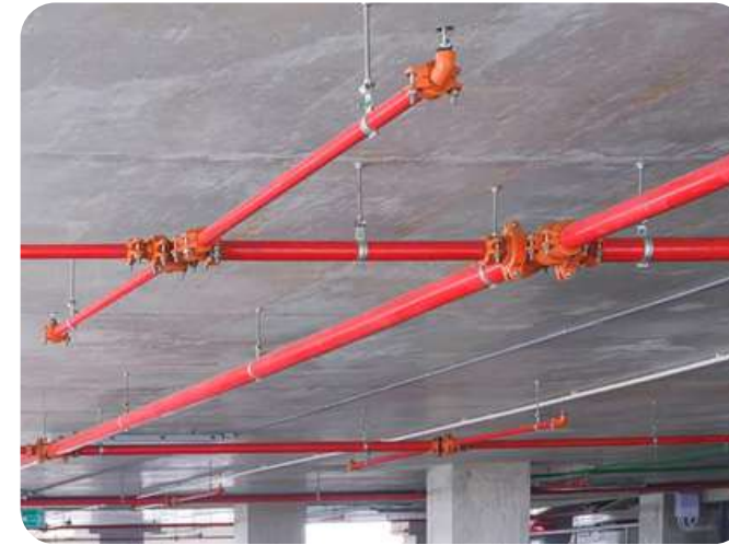
Water Sprinkler System
